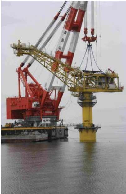
Mating topside to substructure
