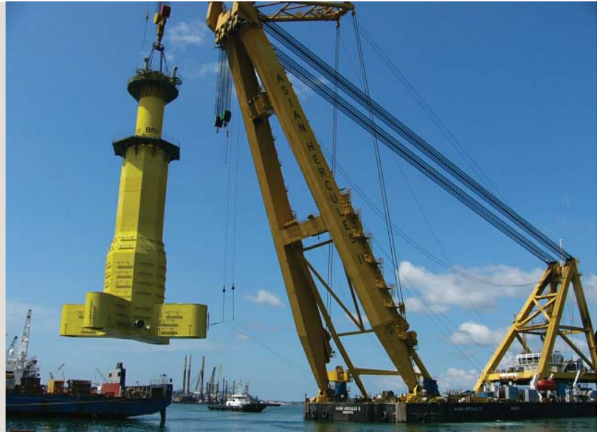
Pile based TLU substructure
