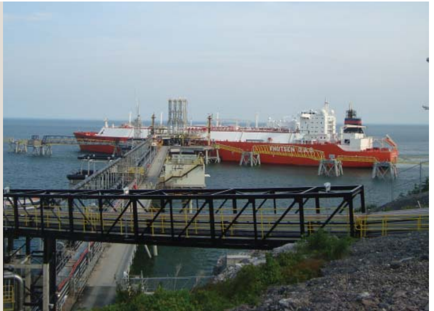
Canaport marine facilities
