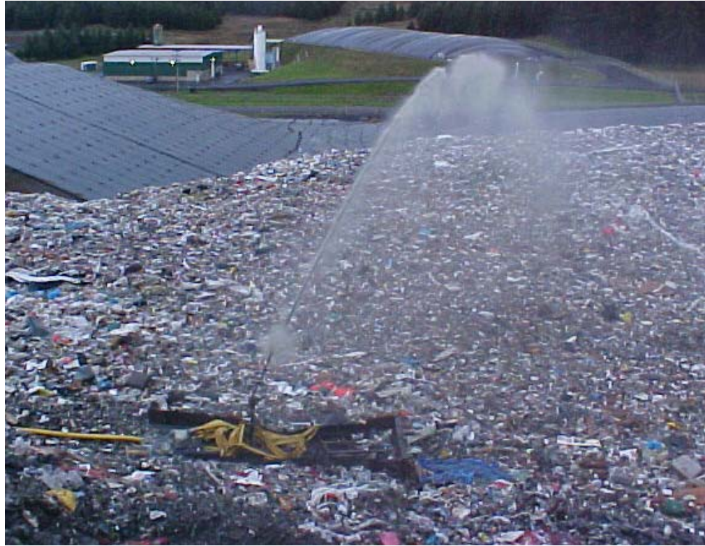
Figure 5. Spray-recirculation of leachate from internal collection sumps onto landfill top lift surface for accelerated bioreactor decomposition of organics.
