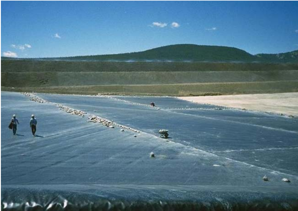
Figure 9. Unsupported toe of leach pad expansion base liner for external solution gravity-flow. Operating heap stack in background with benched slopes and surface spray leaching.
