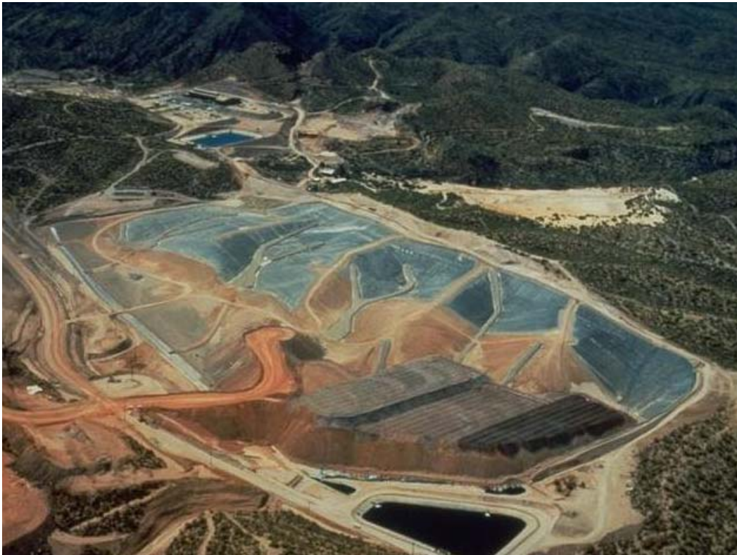
Figure 1. Heap leach operation showing base liner in background, drain placement in canyon bottoms, ore stacking in middle, leaching in bottom right and gravity flow to external ponds.
