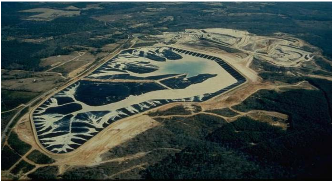
Figure 4 – Conventional above ground lined tailings impoundment contained by a compacted earthfill dam embankment in South Carolina, USA. Perimeter pipeline tailings slurry disposal is shown above the geomembrane liner with an interior water pool pumped in a water return pipeline back to the plant facilities for reuse.
