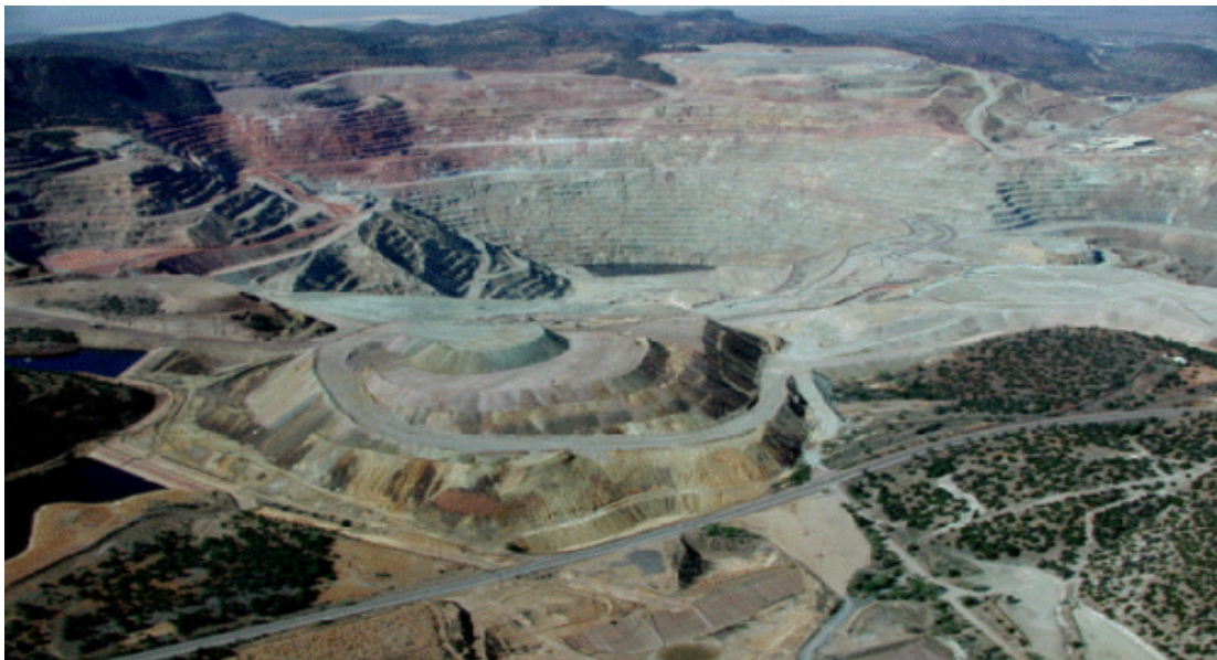
Figure 6 – Lined leach pad constructed in lower left portion of open pit copper mine in 1994. A similar low grade ore heap is shown in the foreground adjacent to the mine pit wall limits.
