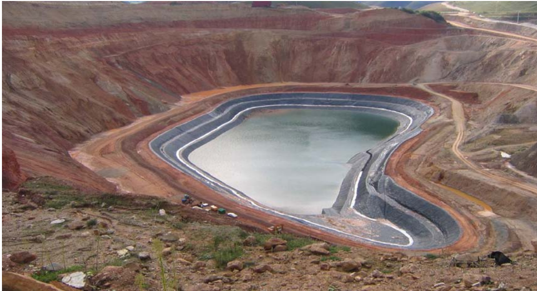
Figure 5 – Lined tailings impoundment for startup conventional tailings slurry disposal within a depleted open pit gold mine in Northern Spain
