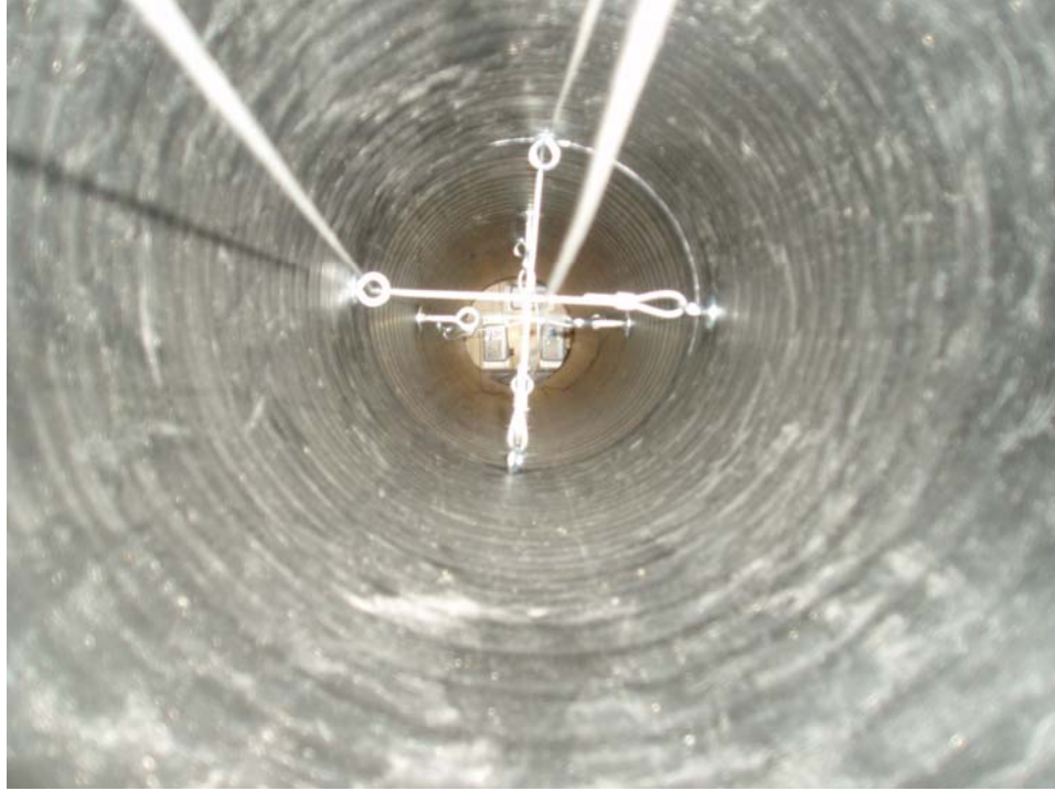
Photo 2 - Deflection Measurement System Before Test
