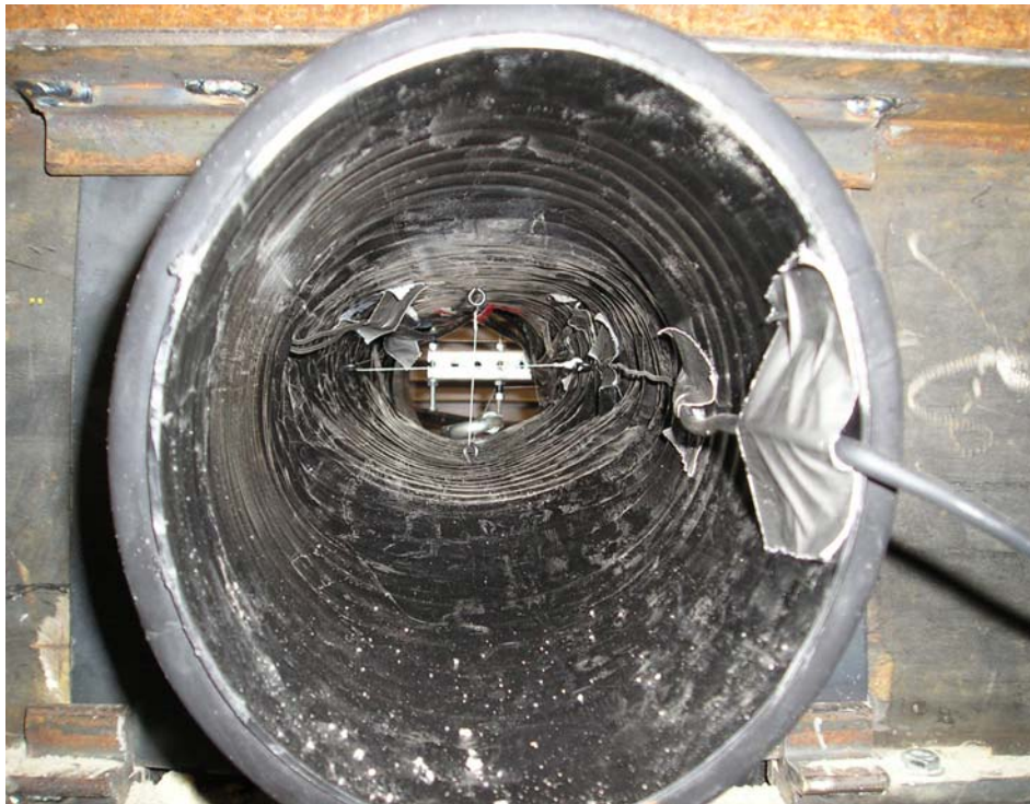
Photo 3 - Pipe Deflection at Maximum Load for Series C
