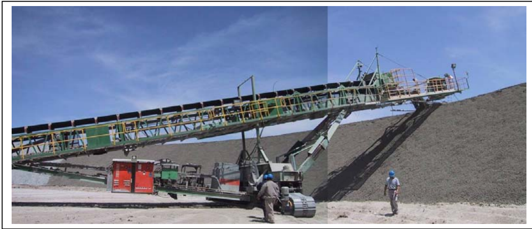
Figure 3.4 Radial Stacker Operating in Retreat Mode, Chile
