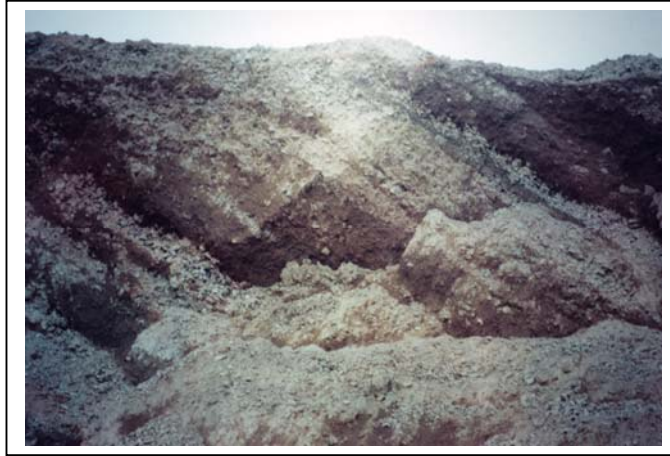
Figure 3.2 Segregation and solution channeling in a lateritic heap trigger a large slope failure
