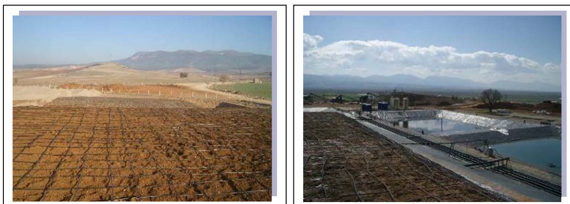
Figure 3.8: Çaldağ Pilot Test Heap during Operation
