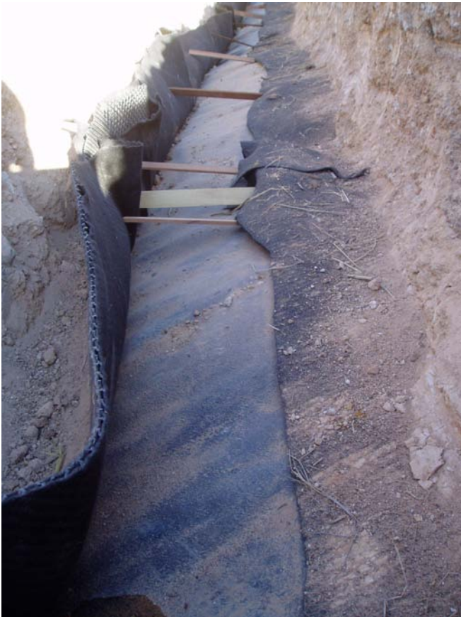
Figure 2. Perimeter trench with geocomposite separation.
