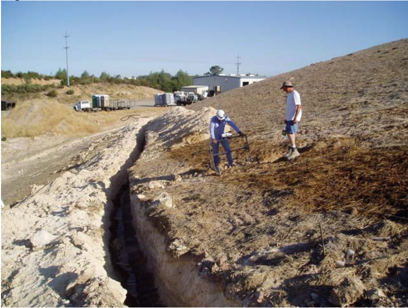
Figure 2. Perimeter trench with geocomposite separation.
