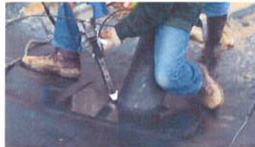
(d) Welding the pipe to the plate. Ideally another welded boot will be installed over this.
