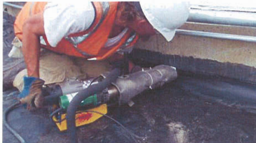
Figure 16. Welding geomembrane to embedment strip with preheater on extrusion gun.
