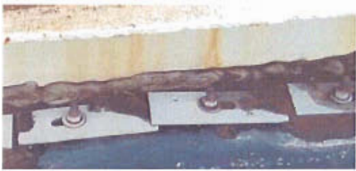
(c) Hairline crack in concrete will defeat batten when submerged.
