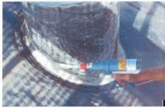
(f) Conducting hand-held spark test on boot weld.
