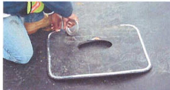
(b) Applying aluminum tape to bottom of plate for spark test.
