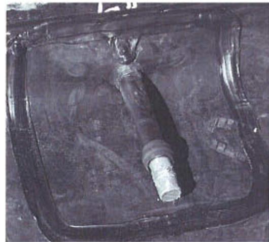
(b) Installed penetration.
