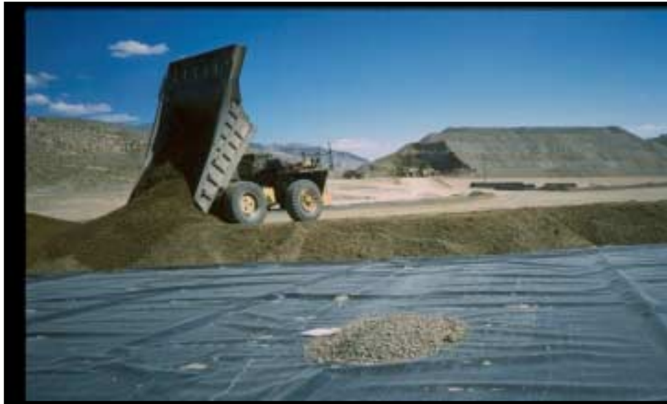
Photo 2 – Placement of Drain Cover Fill on Leach Pad Liner (Nevada)
