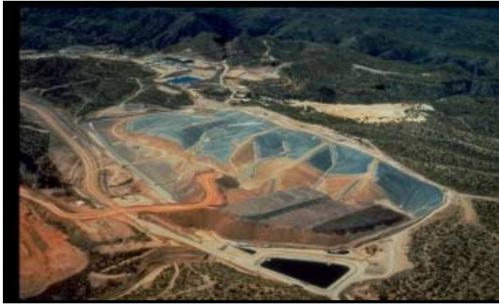
Photo 1 – Stacking and Leaching of Ore Heap on Lined Leach Pad (Arizona)
