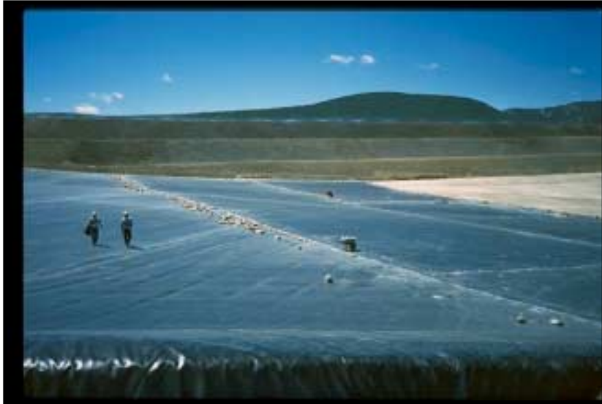
Photo 5 – Lined Expansion of Leach Pad for Heap Operations (Montana)
