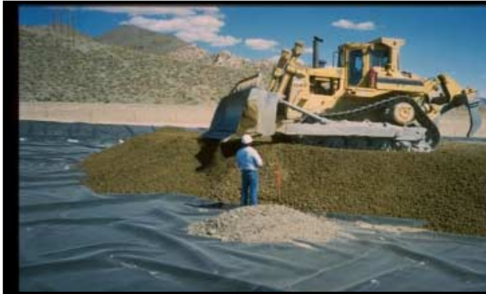
Photo 3 – Dozer Spreading Drain Cover in Controlled Lift (Nevada)
