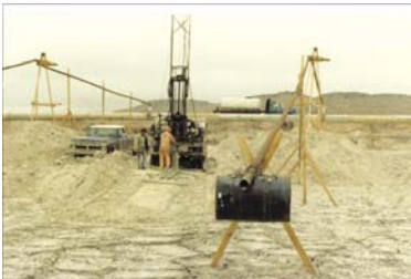
Fig. 1: Tailings beach geotechnical investigation for dam raise
