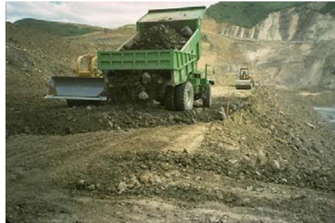
Fig. 8: Rock fill shell construction on steep slope
