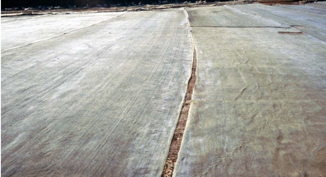
Photo 1 - Observed Field Separation of GCL Overlaps
