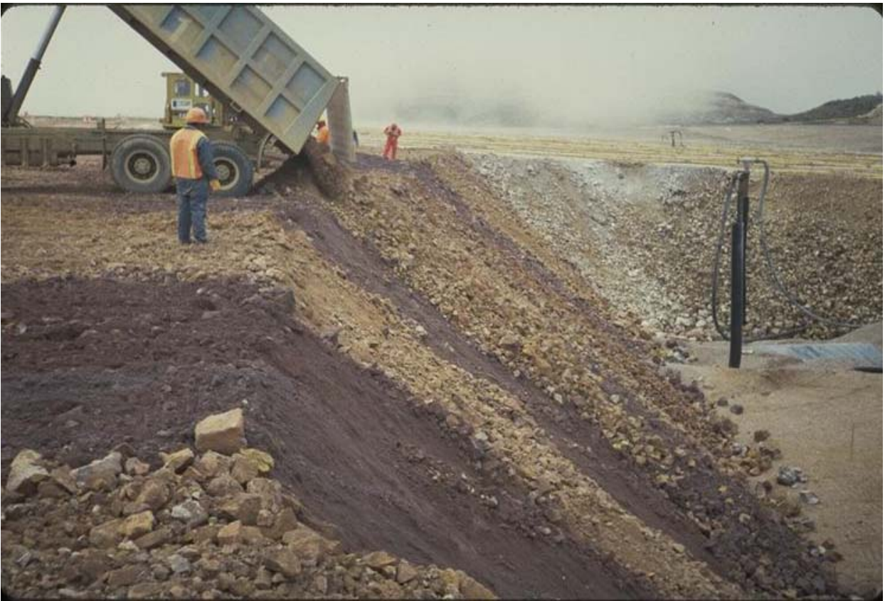
Photo 2 – Earthfill and Rockfill Placed in Controlled Fill Lift Thickness
