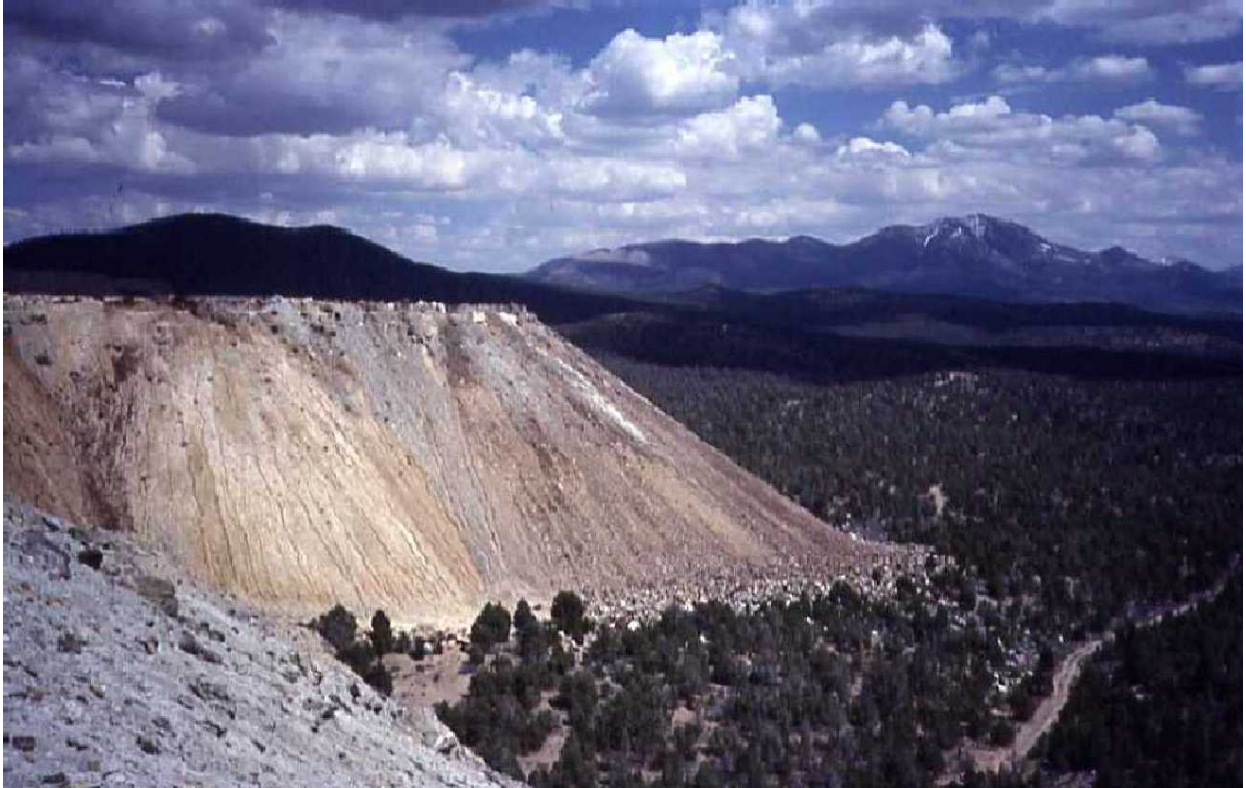
Photo 3 – Predominantly Earthfill Waste Dump with Boulders at Downhill Toe
