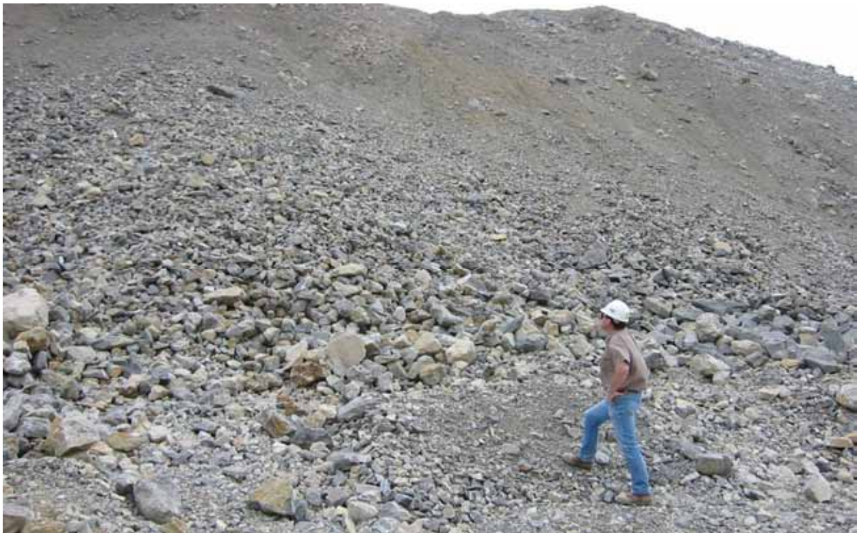
PHOTO 2 – SMALLER ROCKFILL FRAGMENTS AT TOP OF BORROW STOCKPILE TRANSITIONING TO LARGER ROCKFILL FRAGMENTS AT BOTTOM
