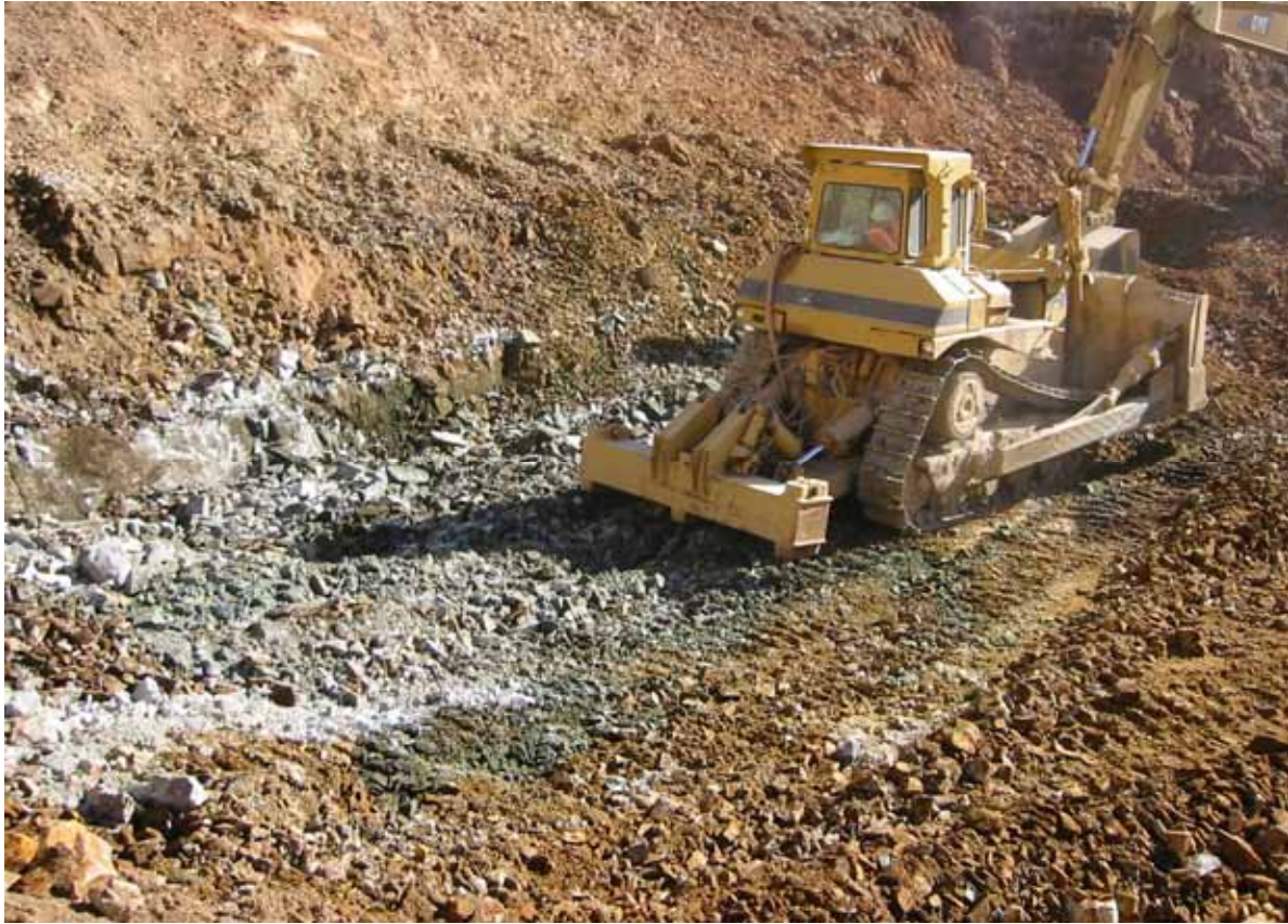
PHOTO 5 – ROCK EXCAVATION USING A DOZER WITH SINGLE RIPPER TOOTH
