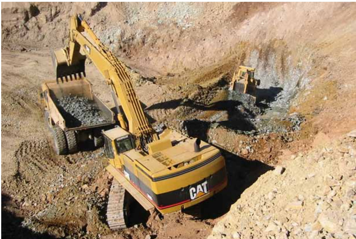
PHOTO 6 – RIPPED AND DOZED ROCK MATERIALS LOADED INTO HAUL TRUCK
