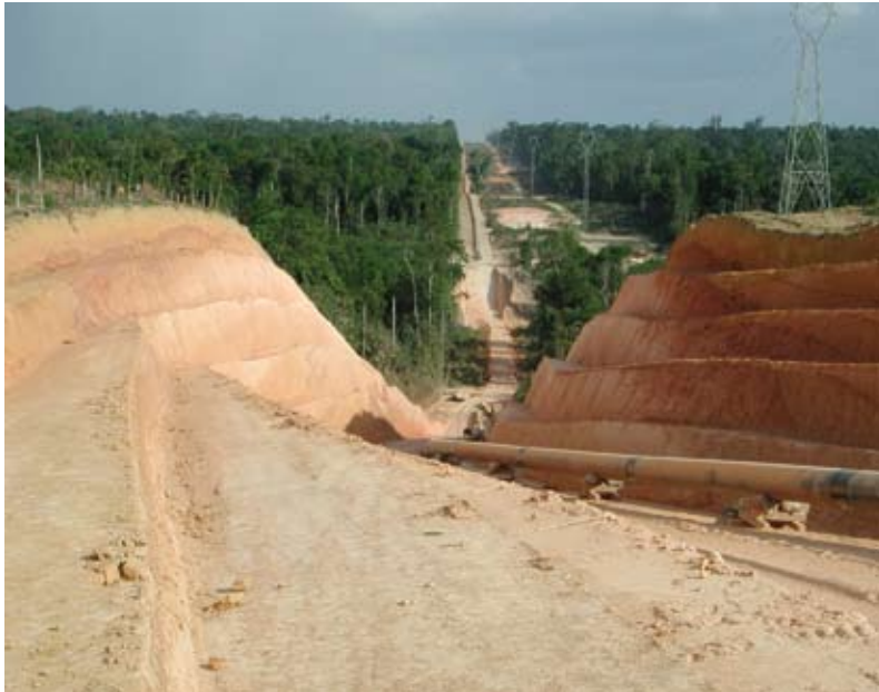
Above Slurry pipeline construction
