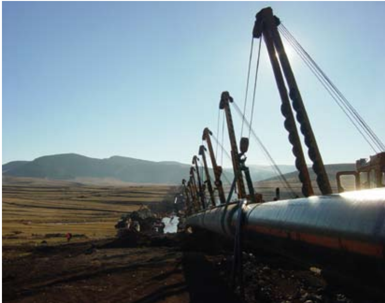
Above Crude oil pipeline construction
