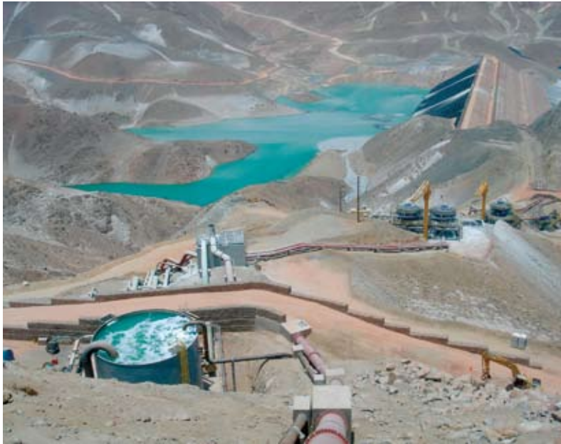
Above Copper tailings cyclone dilution tank and cyclone stations
