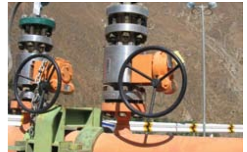
Top Pipeline control room
