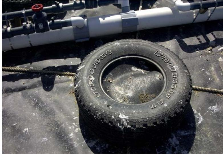
Figure 5. Photo of Tire Protection Over Sandbag.
