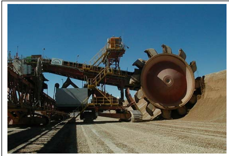
Figure 3.6 Reclaimer Bucket Wheel, Chile
