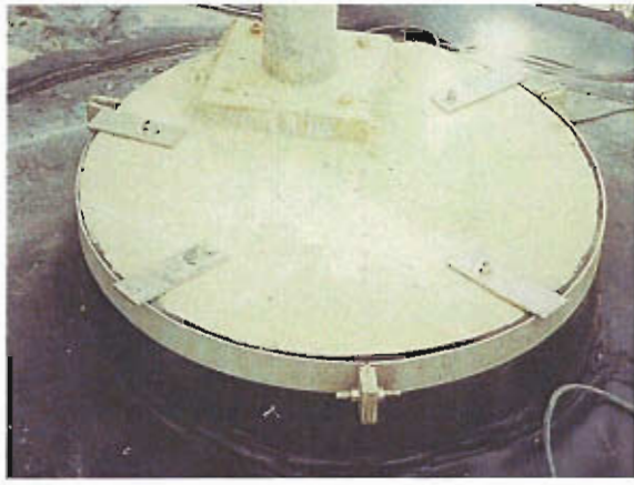
(d) Heavy wide custom clamp around end of a penetration.
