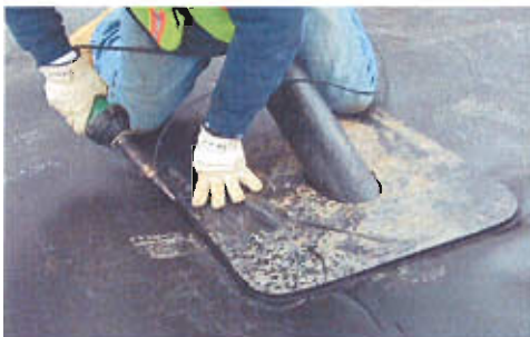
(c) Heat-tacking the plate to the free-field geomembrane.
