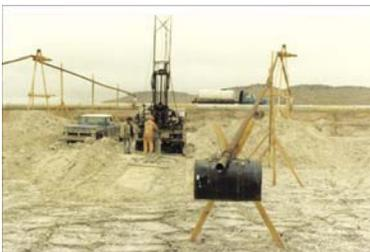
Fig. 1: Tailings beach geotechnical investigation for dam raise
