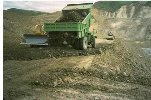
Fig. 8: Rock fill shell construction on steep slope
