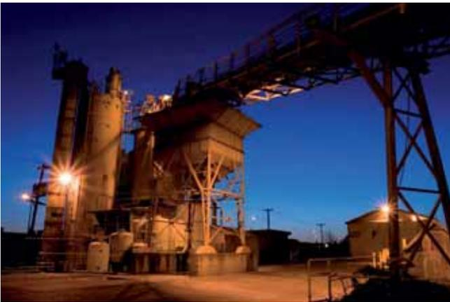
This project involved an initial study of backfill options, followed by the design and construction management of a surface cement slurry plant and pumped reticulation system, as well as the underground cement slurry/aggregate dosing and mixing system.
