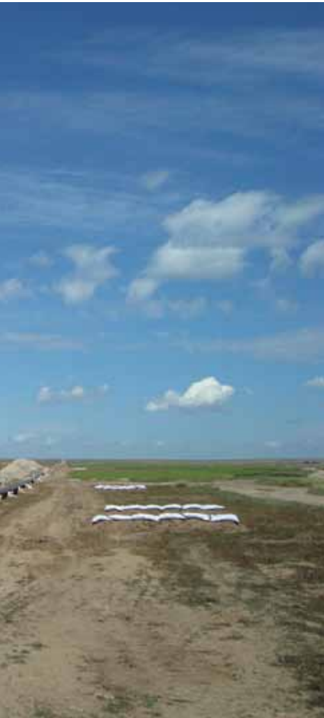
Bao Tou (Bai Yun E Bo) Iron Concentrate, Water and Thickened Tailings Systems, under construction, China
